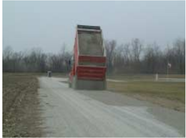
The dump truck drivers spread the rock as they unloaded it, and did a pretty good job!
